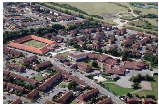
Shinewater Community Centre
